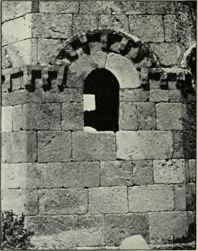
FIG. 264.—Ana Tepessi, detail of apse.
